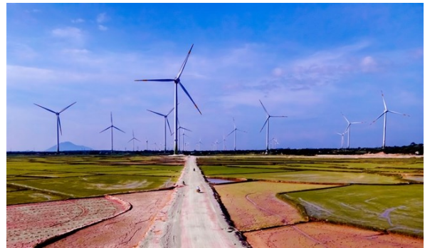
A wind farm of Trung Nam Group in Ninh Thuận Province
