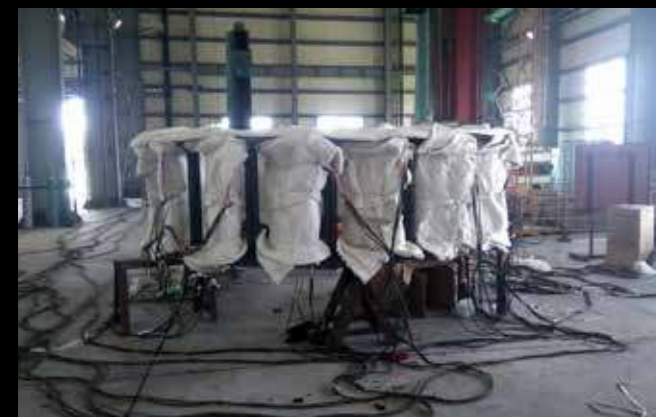
Induction heating for preheating
