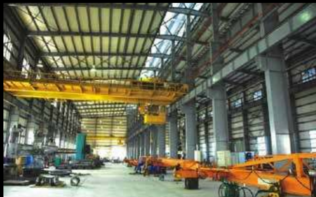
Indoor workshop (Area: 12,000m 2 )
