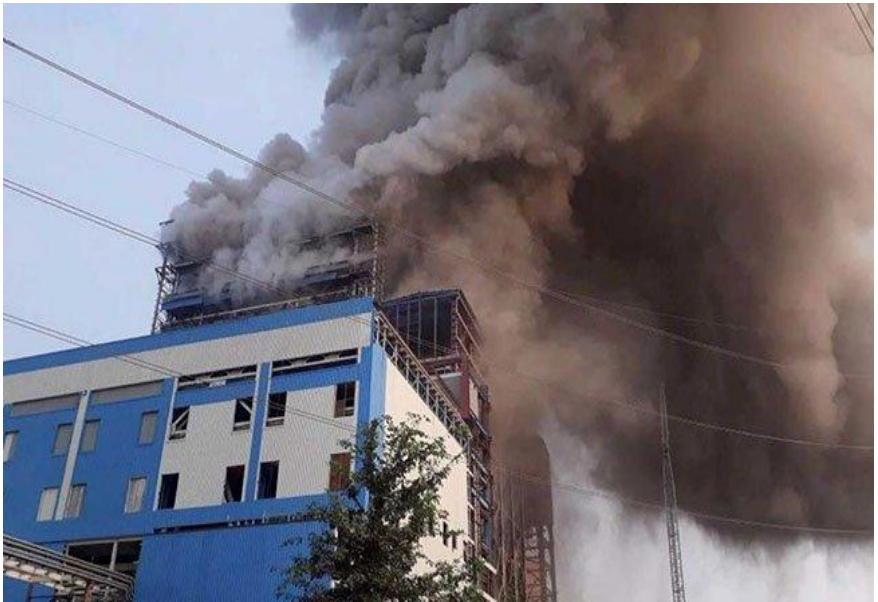
Smoke from the boiler explosion in India, 01-11-2017.
